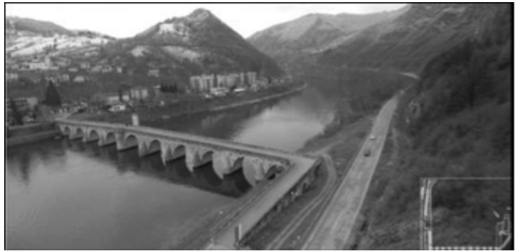
Bridge Prior to Restoration Implementation Works (KGM Archive)
