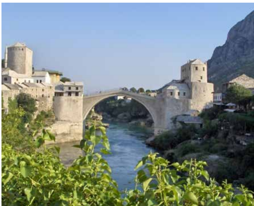
Bridge after Restoration Implementation Works (KGM Archive)
